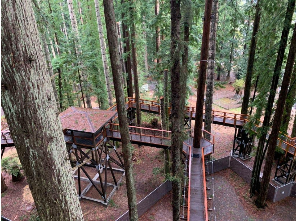
Skywalk and platforms around trees
